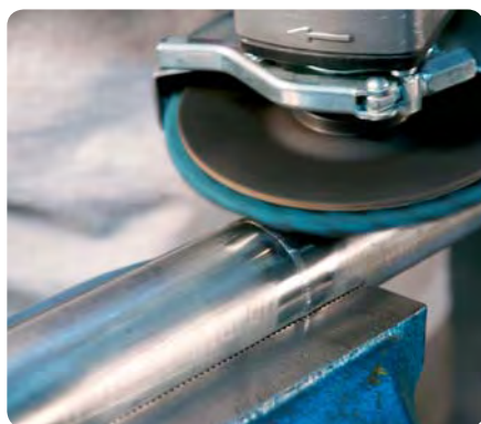
Grinding thin welding seams and removing thermal bluing
